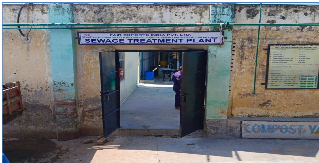
Figure 16: Sewage Treatment Plant
